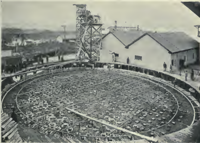
Concrete Pile Foundation for a thirty thousand barrel oil storage tank.
